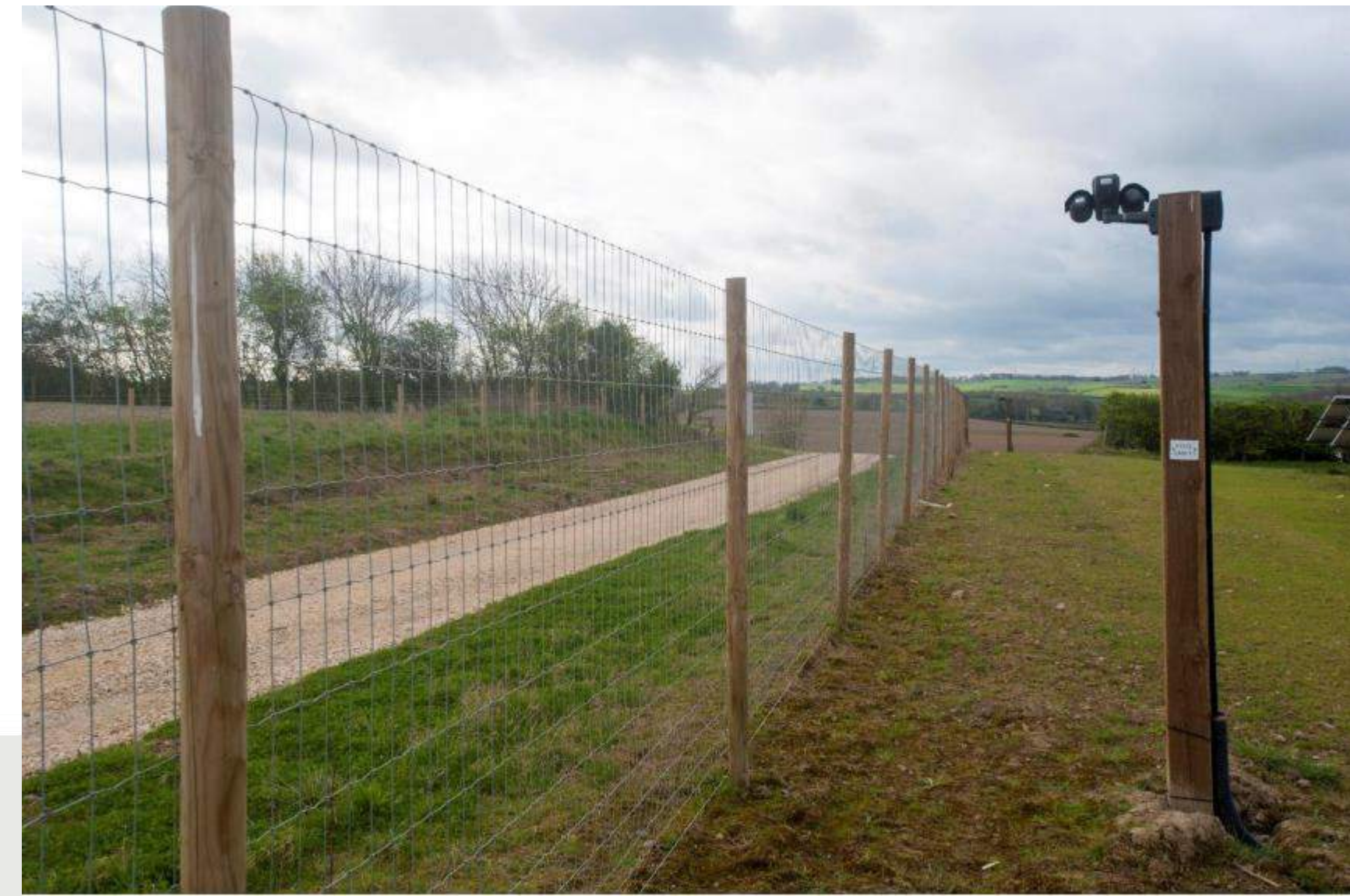
Fencing, CCTV, Access tracks
